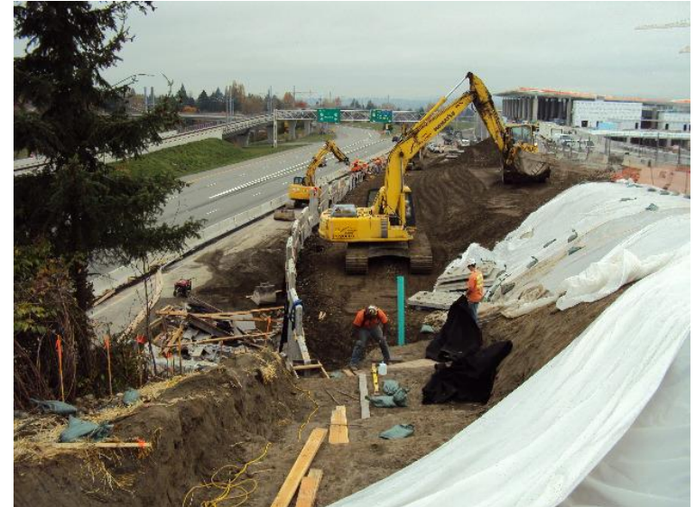
CRCF ORI 518 On Ramp SEW Wall
