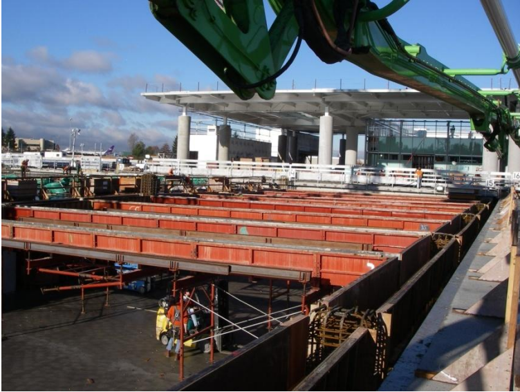
Form Installation – Area F – Last Placement Area
