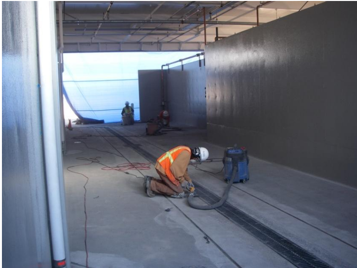
QTA #1 – Car Wash Bay Substrate Preparation
