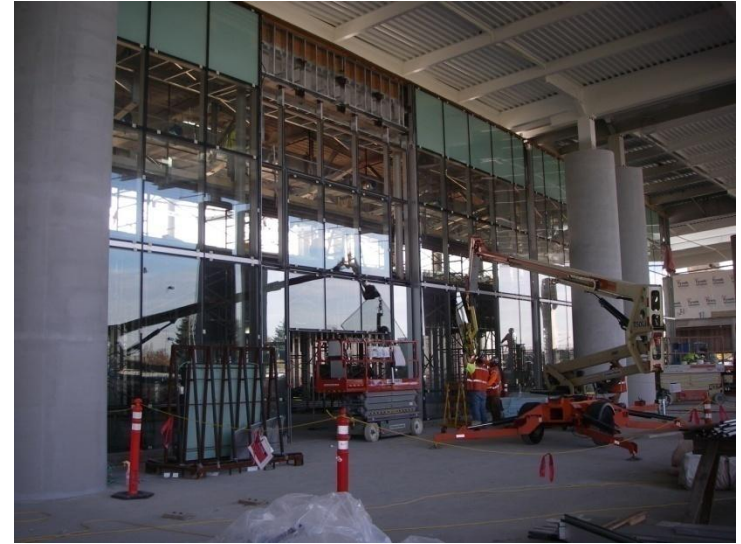
CSB Curtain Wall Glazing in Progress
